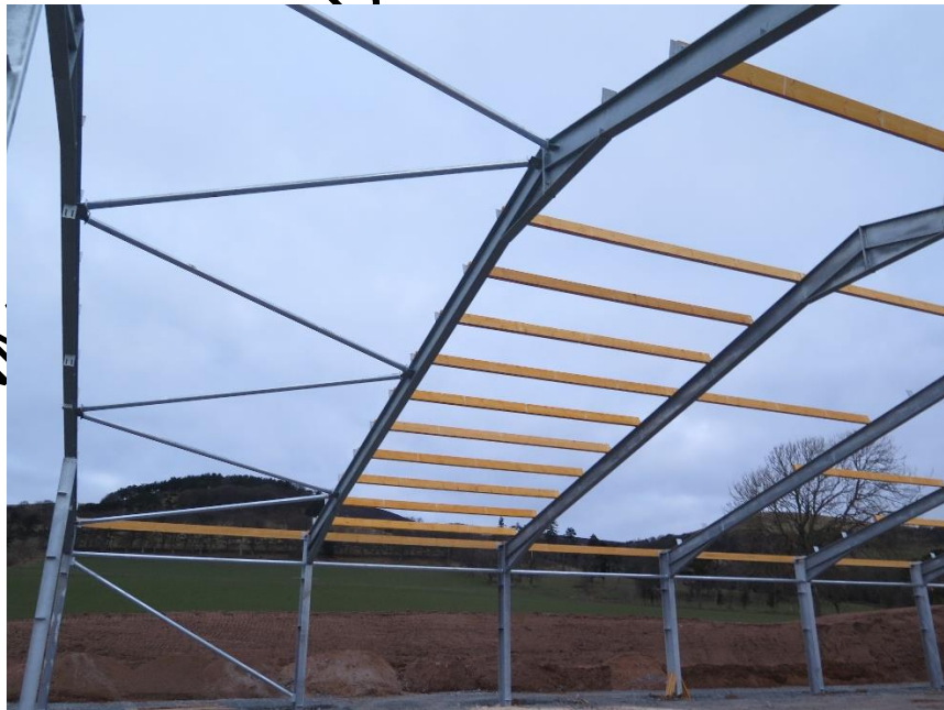
Steel portal frame construction progress
