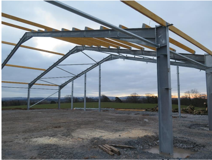
Steel portal frame construction progress
