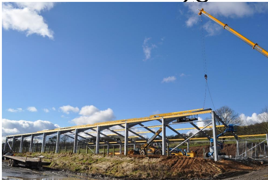
Steel portal frame construction progress
