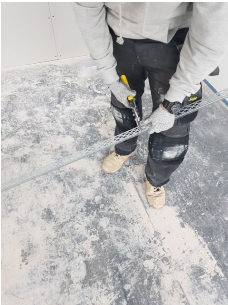
Photograph 18: Showing accuracy in cut to the dimensions for thin coat angle beads fixing (prior to positioning)
