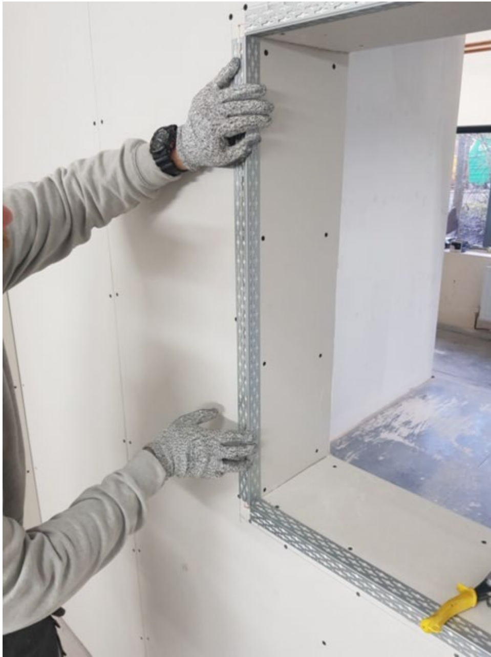
Photograph 21: Showing accuracy of all positioned beads
