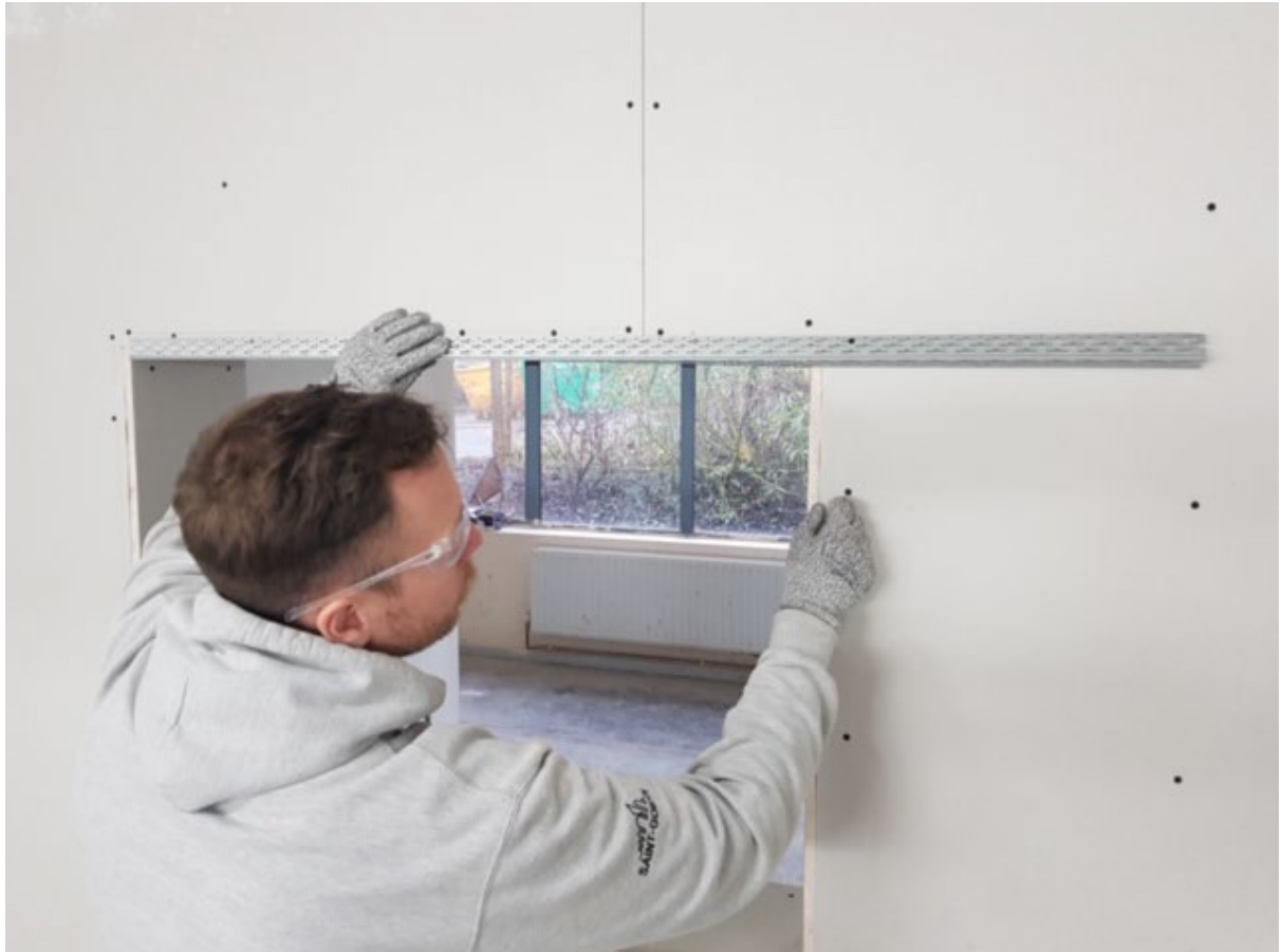
Photograph 19 - Showing pre-positioning of beads
