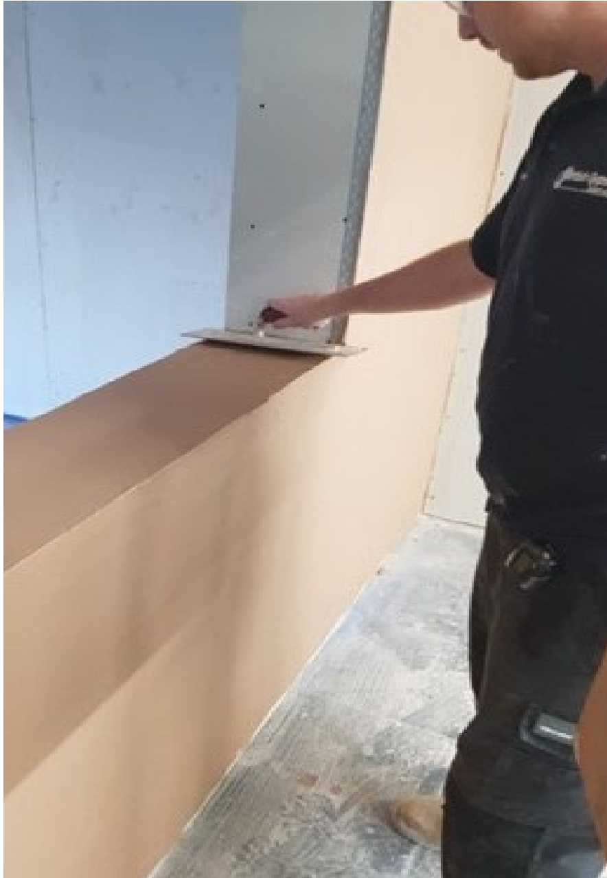
Photograph 26 - Showing plaster application in production
