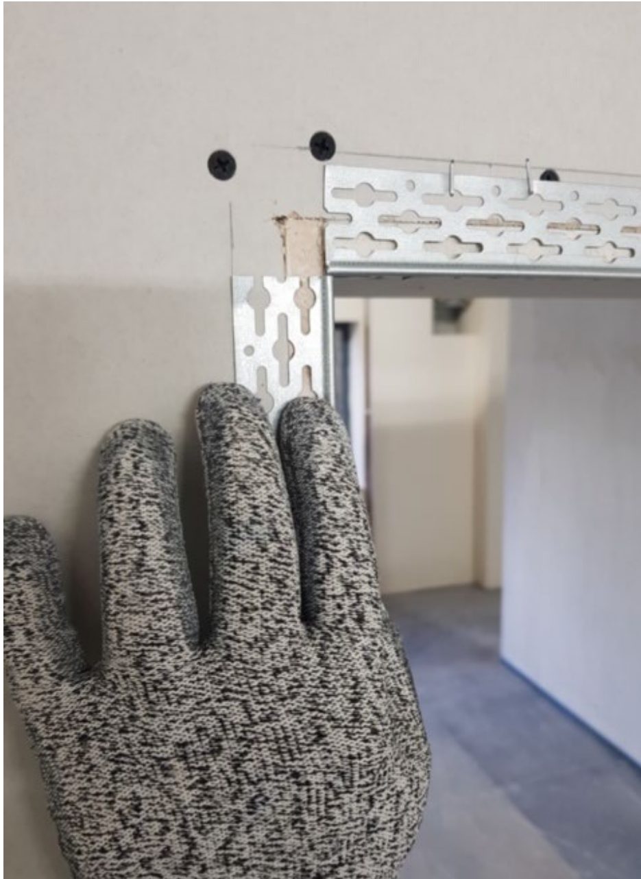
Photograph 20: showing positioning of beads
