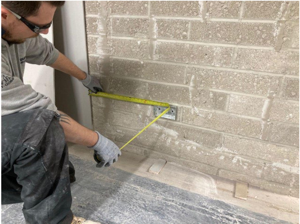
Photograph 2 – Showing accurate service box measurements for transfer to plasterboard.
