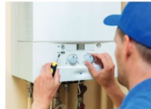
▲ Figure 3.17 Retrofit installer fitting an energy-efficient boiler
