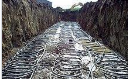
A horizontal slinky loop prior to being covered with soil.
