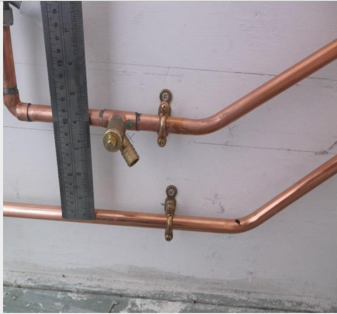
Task 2 Photo ref 11. Pipe centres to design brief 100mm centres. Munson clips not aligned.
