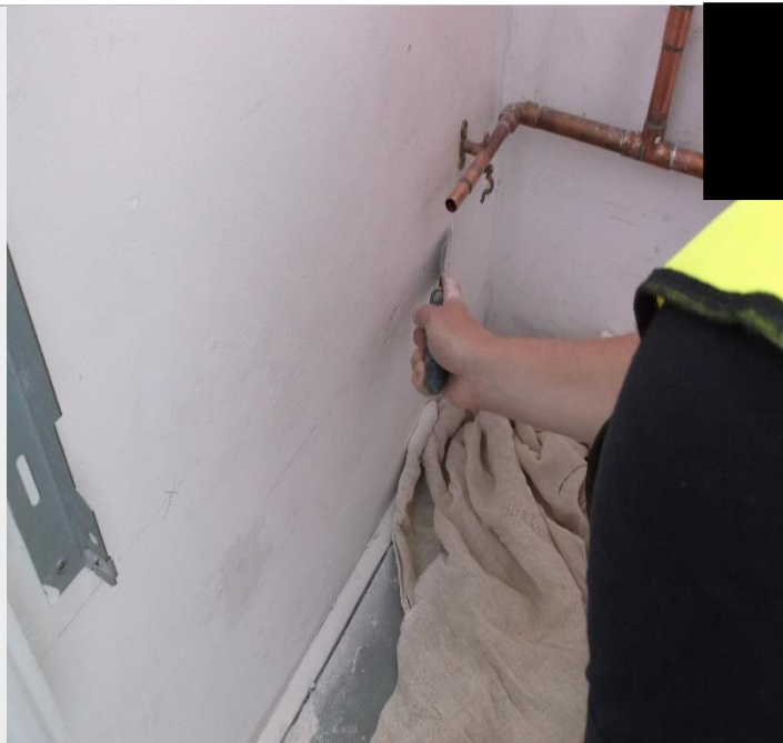
Task 2 Photo ref 26. Filing the holes with decorating caulk.
