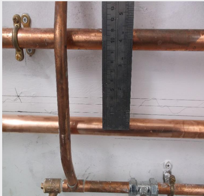
Task 2 Photo ref 12. Pipe centres as to design brief 100 mm centres.
