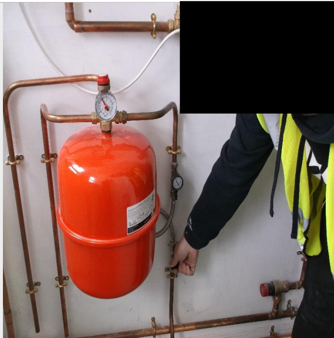
Task 2 Photo ref 16. System filled to 1.5 Bar test pressure
