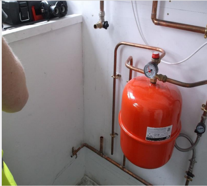
Task 2 Photo ref 1. Installing the magnetic filter.
