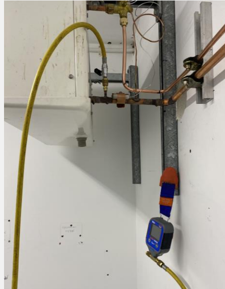
(Photograph 11) Vacuum pump and Torr gauge showing correct connections with Torr gauge at furthest point from vacuum pump
