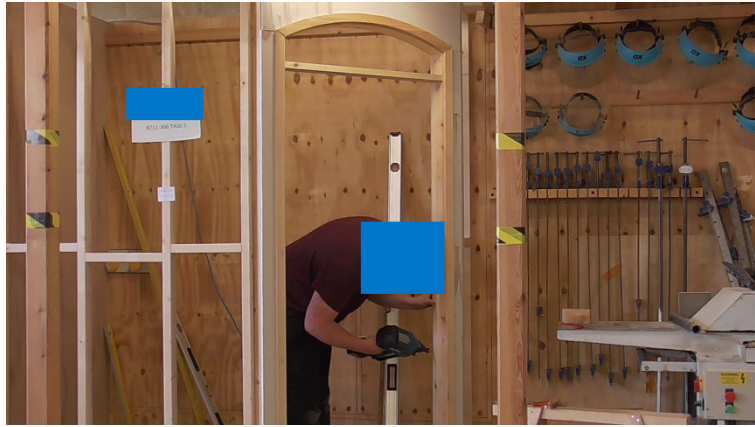
Fitting doorstop before offering the door into the opening
