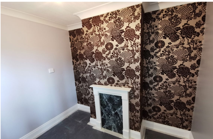
Photographs 16 showing finished wallpaper with detail on drop pattern
