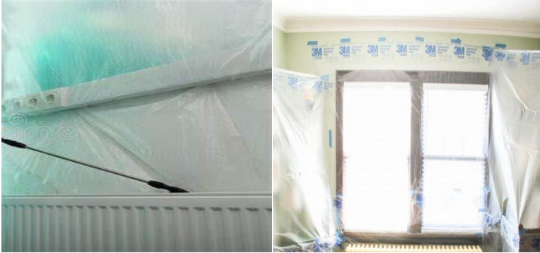
Photographs 24 – 26 showing the preparation/set up and testing of HVLP
