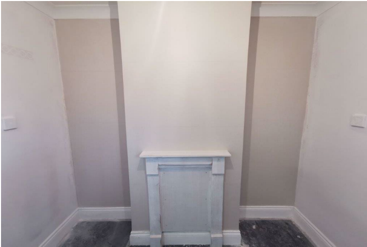
Photograph 8 – showing completed lining paper on fireplace wall
