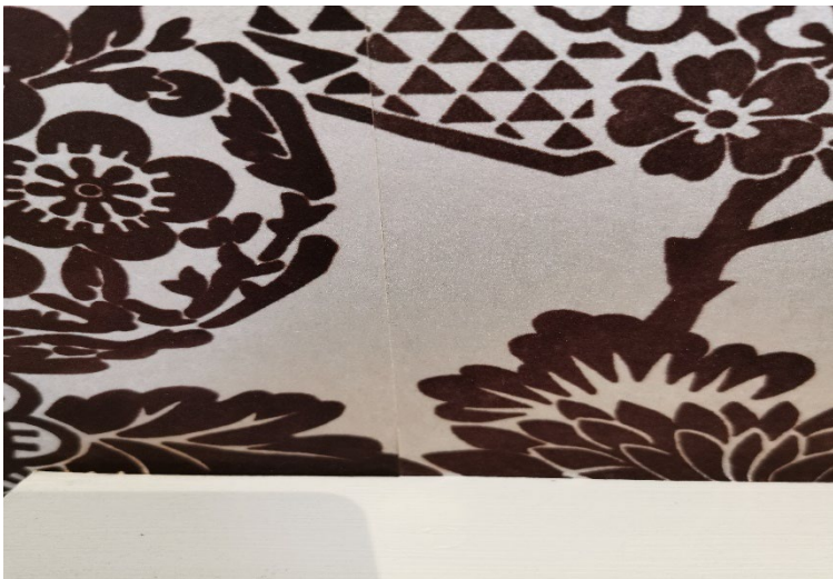
Photograph 11 – showing matching/pattern alignment on wall
