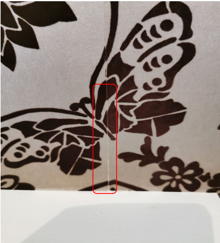
Photograph 14 showing slight gap in one length
