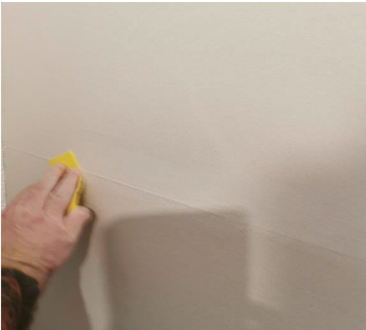
Photograph 9 shows dry edge requiring rectification
