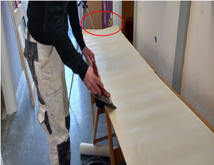
Photograph 7 shows candidate pasting first length of lining paper
