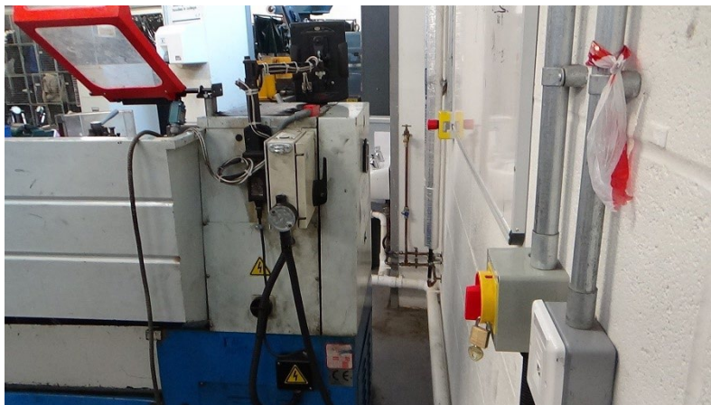
Front panel refitted after maintaining vee belts.
