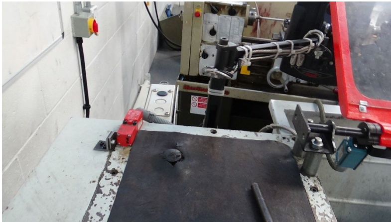
Interlock bracket repaired.
