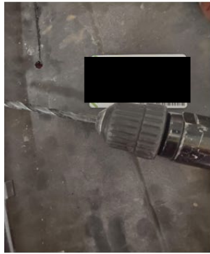
Hole drilled into end of crack.
