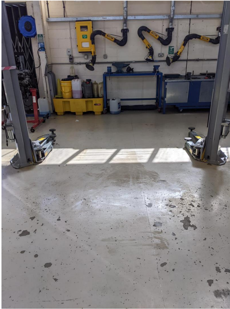
Photograph 4: Photographic evidence shows the two pillar working area reinstated correctly. The area has been cleaned, including an attempt to mop up a spillage – however the floor is still slippery so should include a slippery floor sign.
