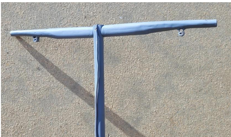
Photograph 12 shows the insulation fitted to the cable fixings.
