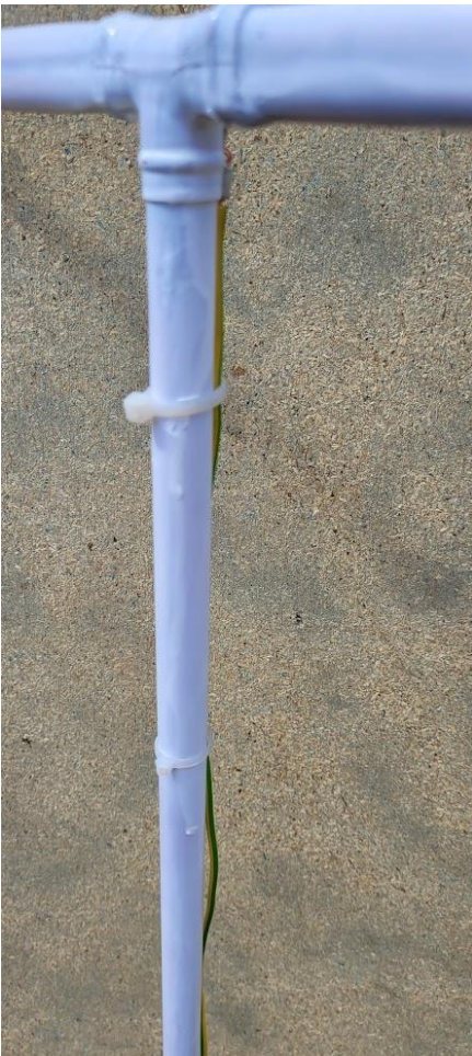
Photograph 13 shows a close-up view of the pylon. The quality of the finish is slightly patchy.
