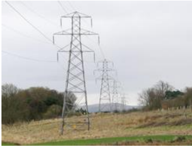
Figure 1: The Milliken Brother's Icon Pylon (source https://www.gorge.org/pylons/structure.shtml )
