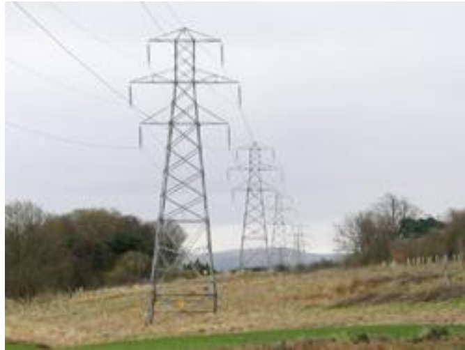
Figure 1: The Milliken Brother's Icon Pylon (source https://www.gorge.org/pylons/structure.shtml )
