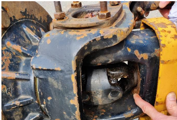
Photo 2 Condition of seals: candidate check after cleaning
